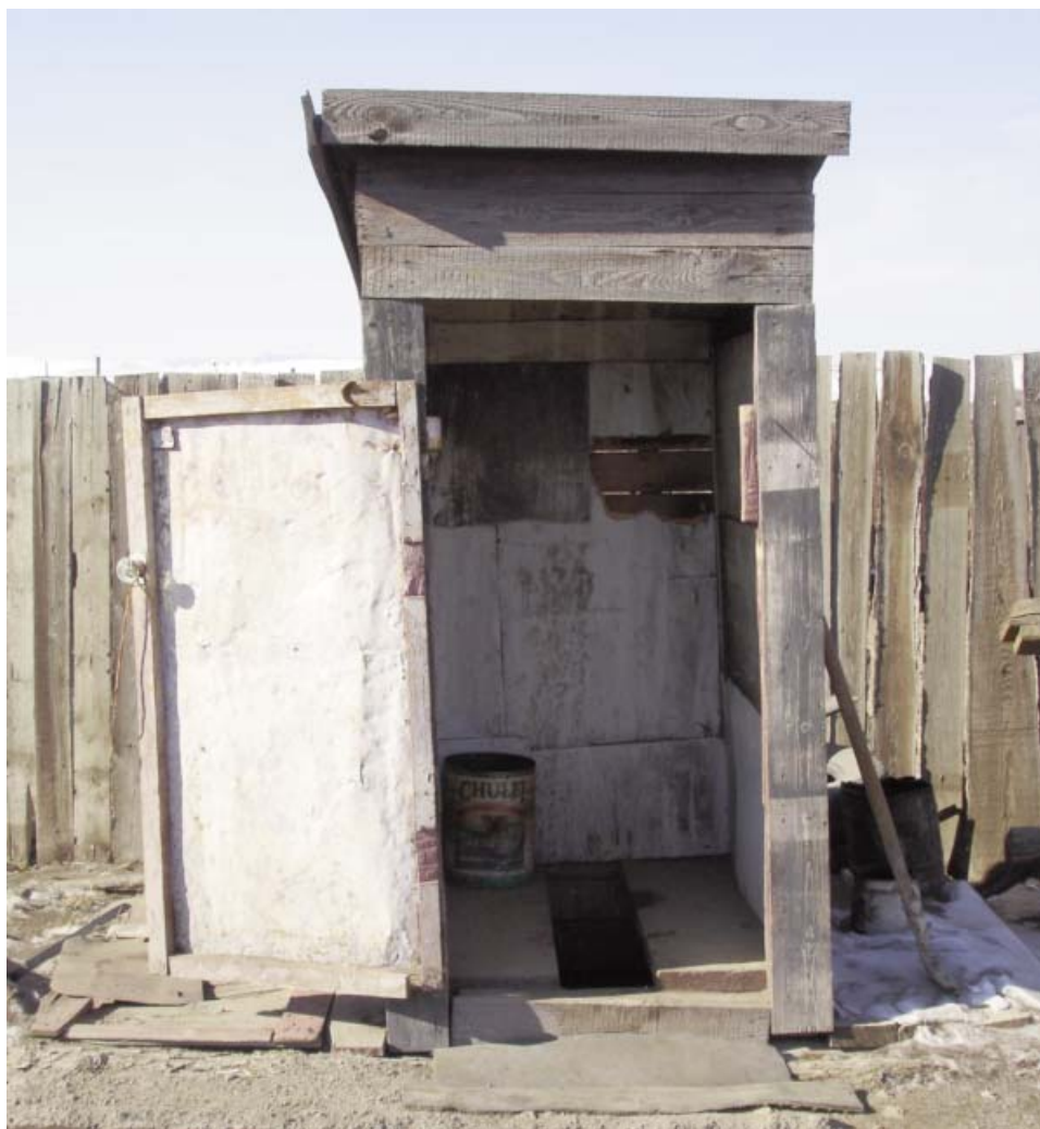
Typical pit latrine
